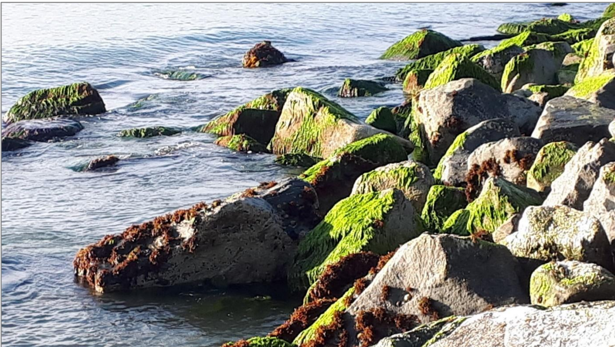
Figure 3.17: Green and brown alge attached to the revetment exposed during low water spring tides at vantage point C
