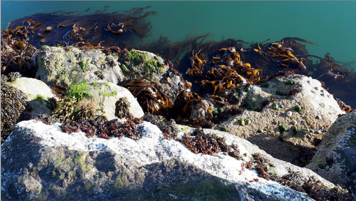
Figure 3.18: Flora and fauna attached to the revetment exposed during low water spring tides at vantage point C
